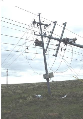
sirens. Several tornados had touched down in the area. One tornado in particular traveled a path from southwest to northeast on the east edge of Lamar. The tornado damaged Lamar Light and Power's electrical distribution system and the
